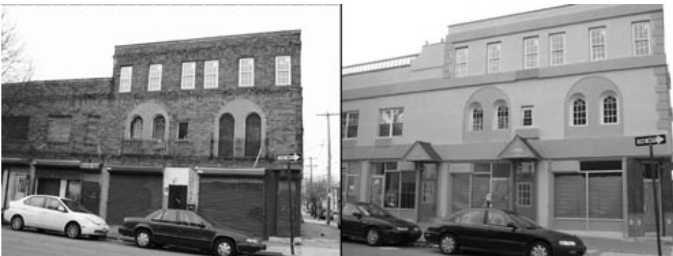
A remarkable transformation: Before, and after
